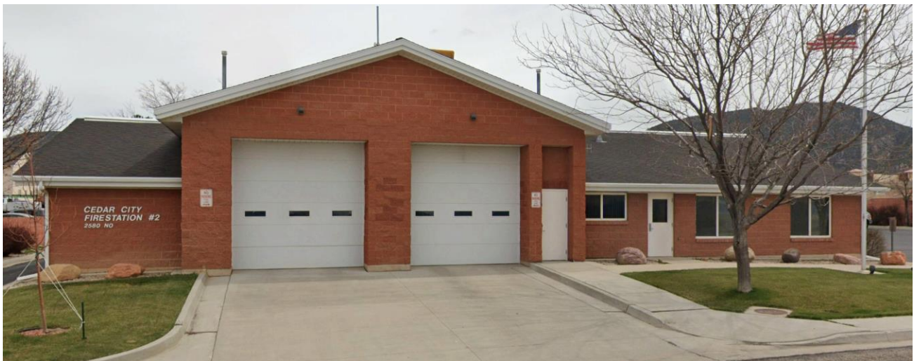
Figure IV-1: Cedar City Fire Station #2
